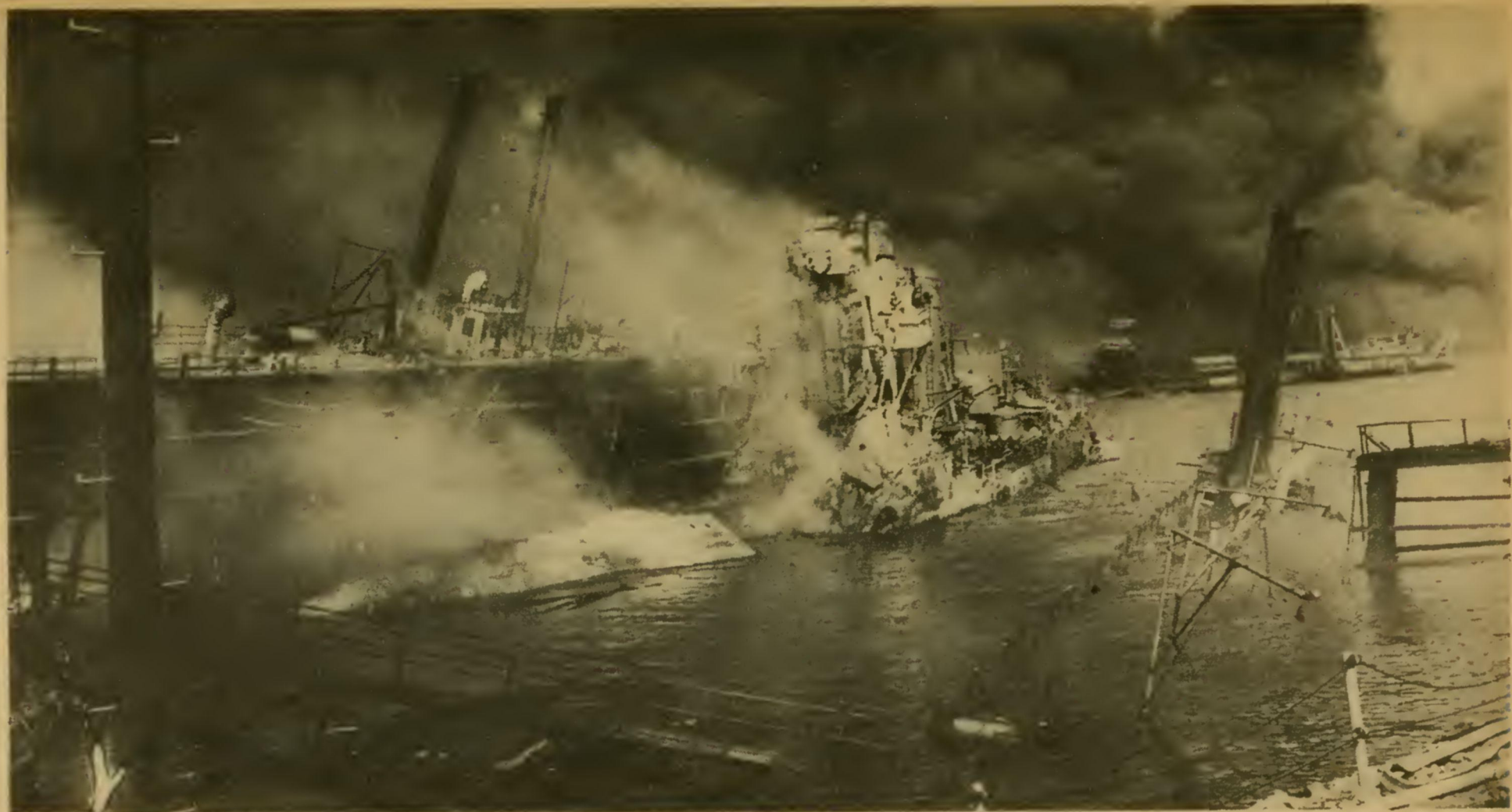
U. S. S. Shaw —Hit by three bombs which exploded her forward magazine, the 1,500-ton destroyer Shaw lies a twisted mass of wreckage in the heavily bombed floating drydock YFD-2. Note the bow of the Shaw lying on its side in the foreground. Part of the drydock, at right, is under water while the other side is listing heavily. Both the Shaw and the drydock are now back in use.
