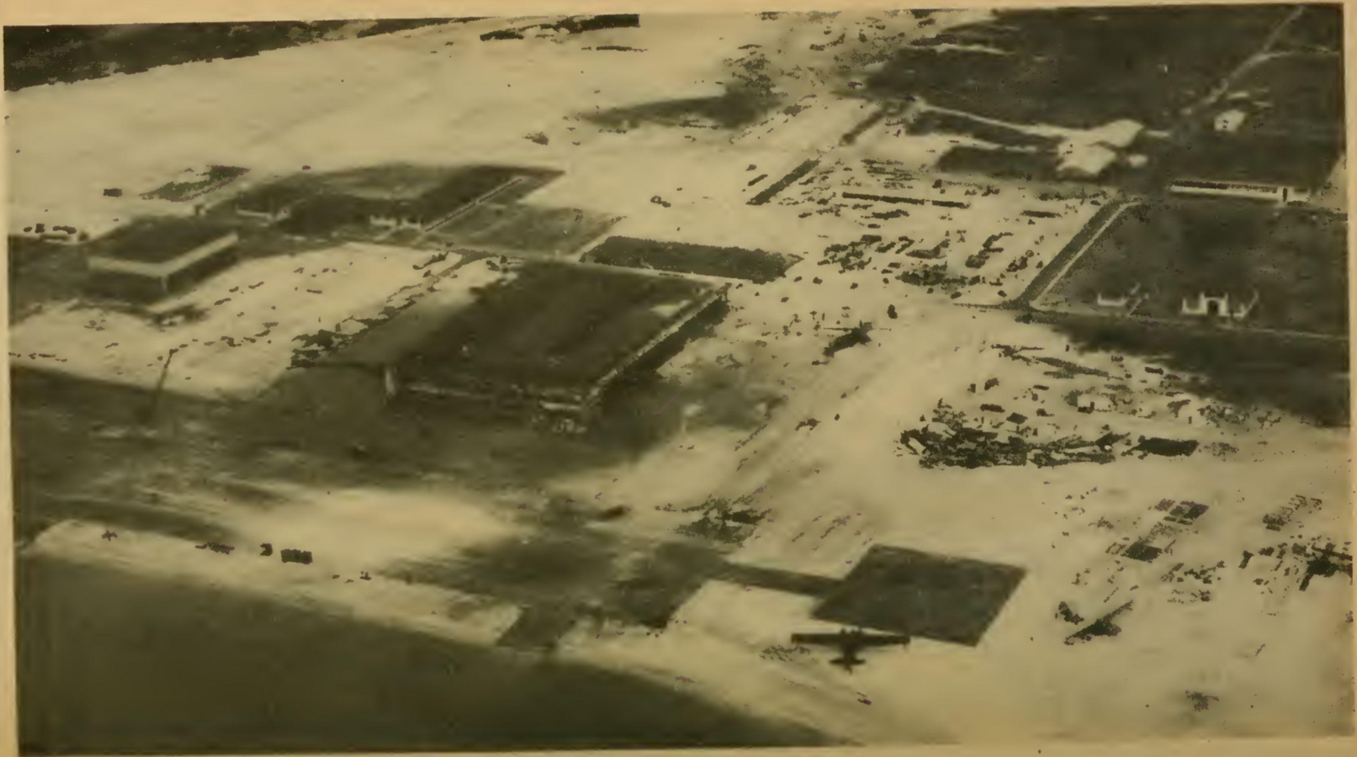
Hangar area at NAS Kaneohe Bay, T. H., showing damage wrought by Japanese bombing attack of December 7, 1941. Altitude 700 feet. Looking northwest.
